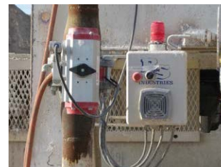
Overflow Warning System
