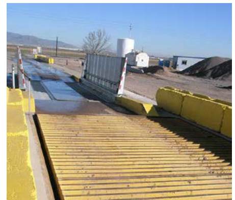
Rumble Grate and Wheel Washer
