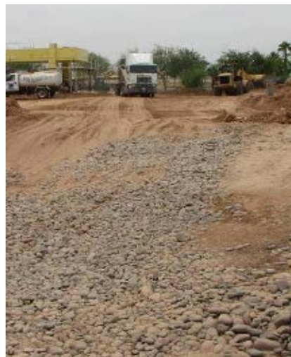
Poorly maintained gravel pad
