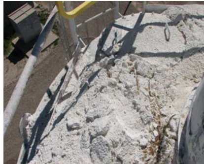
Accumulated Dry Material on a Silo
