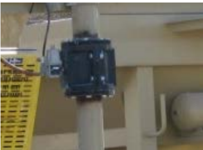
Pressure Control System
